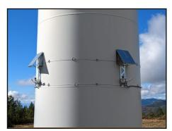
lit is possible to automatically detect and protect against both any type of birds and bats.
