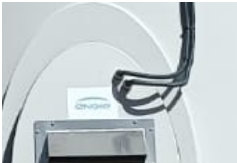
Illustration 8: Wiring through WTG door
