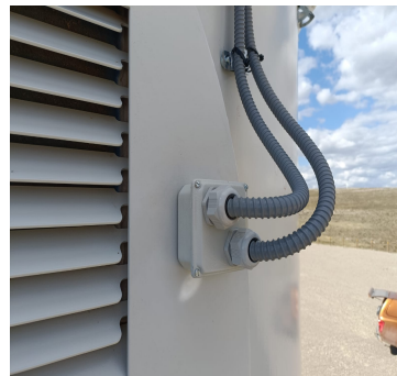
Illustration 9: Wiring through WTG door
