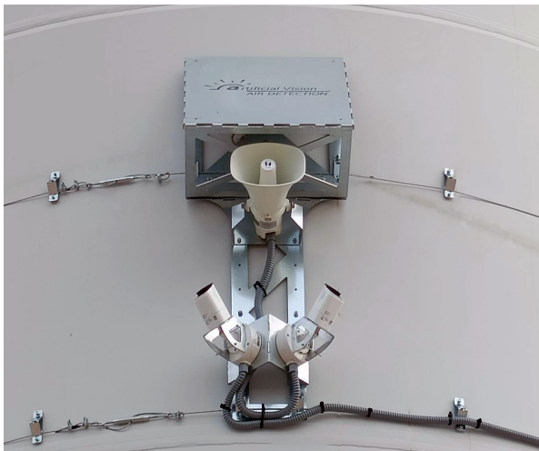
Figure 11: Deterrence module's speaker
