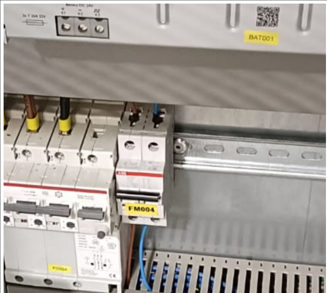
Illustration 7: ArtificialVision power protection FM004
