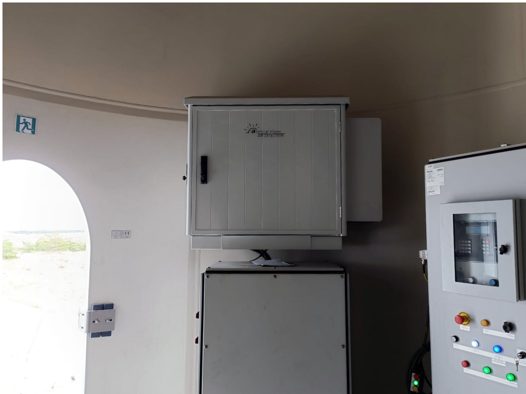
Figure 5: U-Detection rack inside WTG
