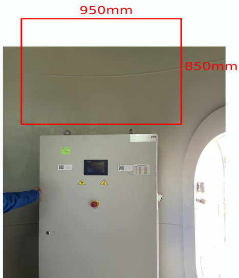
Illustration 3: Installation on the WTG
