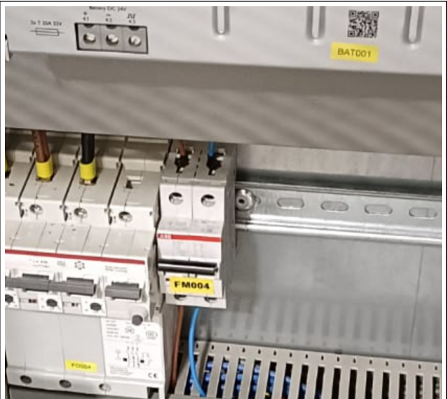
Illustration 7: ArtificialVision power protection FM004
